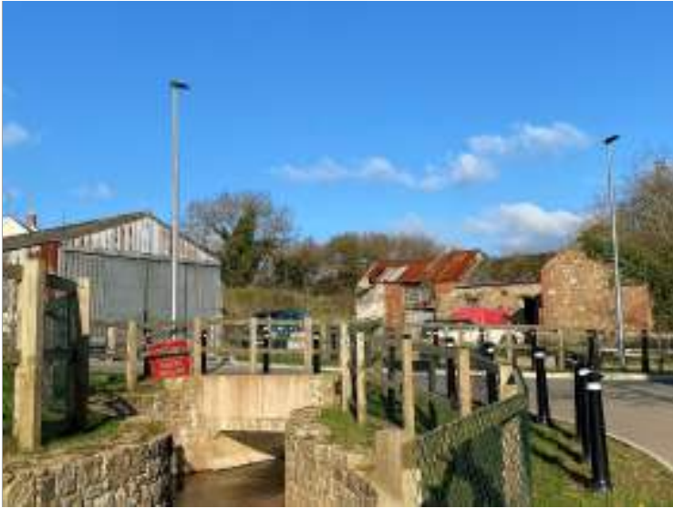
Taken from junction of Rydon Close and Ottery Street with site in background.
